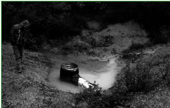
*Water is meant to pond around the sediment riser and deposit accumulated sediment around the riser.*
